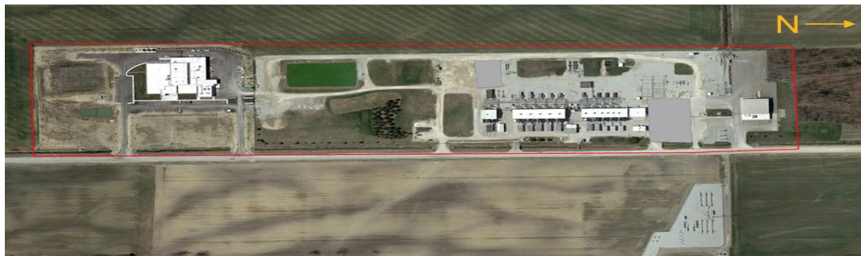
Figure 5: Corunna Compressor Station
