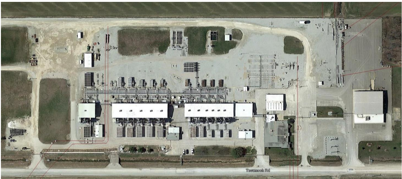
Figure 1.1 Corunna Compressor Station
