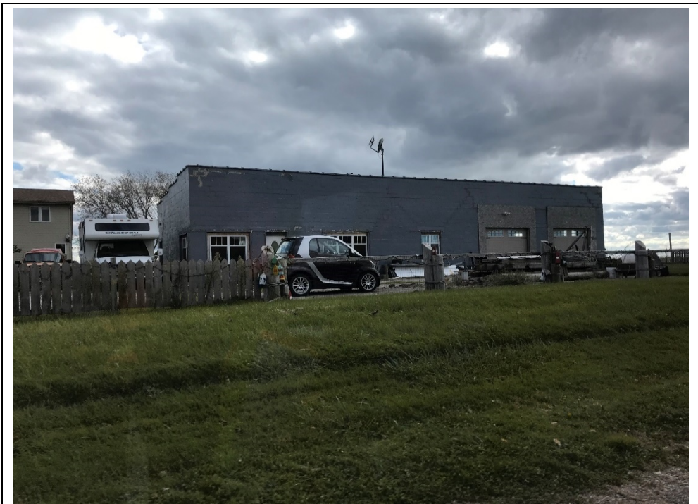
Photo 19 Suspected former garage at Lot 177, south of Talbot Road West, Tilbury East (PSOC 11).
