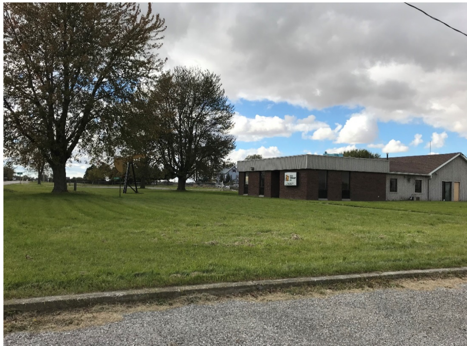
Photo 20 ONCO Petroleum Limited, at 4495 Talbot Trail (PSOC 11).
