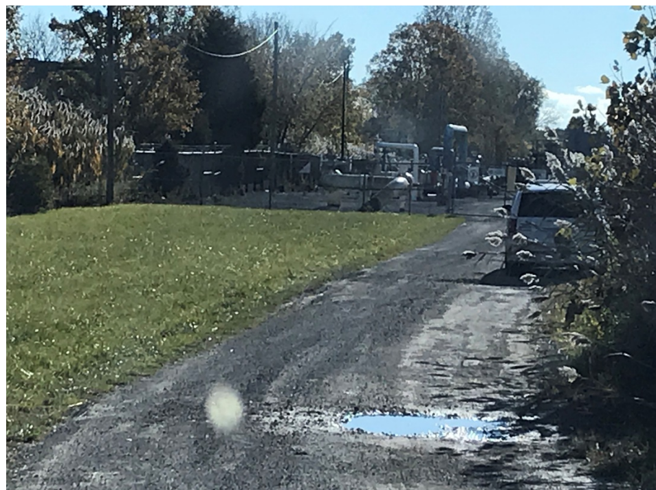
Photo 4 Sandwich Compressor Station, Union Gas Property located at 5100 Concession Road 8 (PSOC 2).
