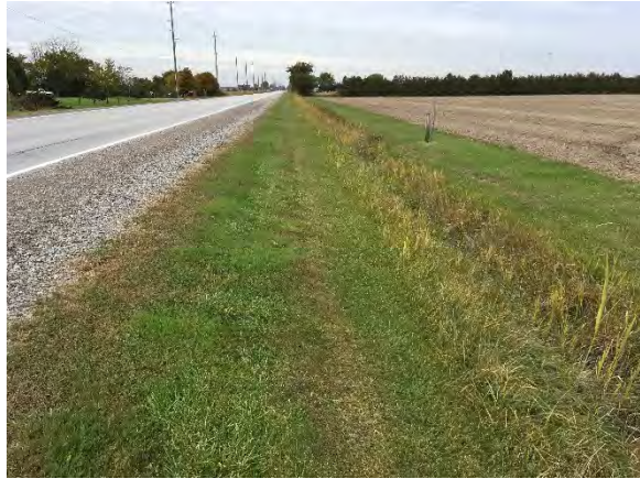
Photo 18: County Road 46 ROW within the Study Area, facing West
