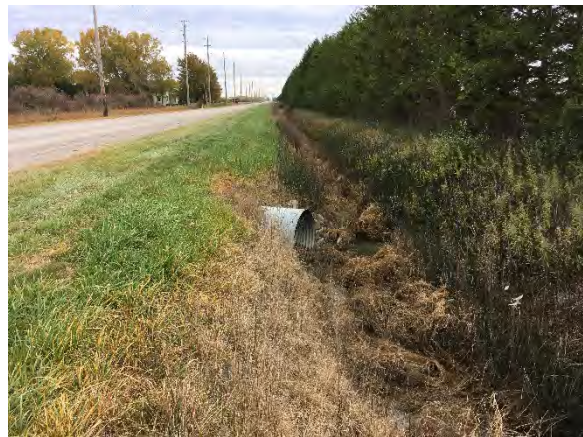
Photo 16: South Middle Road ROW within the Study Area, facing Northeast
