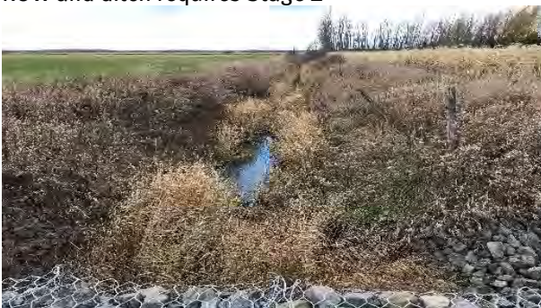
Plate 35: [NW] Channelized creek; Area beyond disturbed ROW and creek channel requires Stage 2
