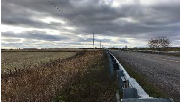
Plate 37: [SW] Burton Road; Area beyond disturbed ROW requires Stage 2
