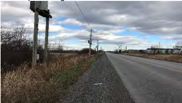
Plate 39: [NE] Burton Road; Area beyond disturbed ROW requires Stage 2
