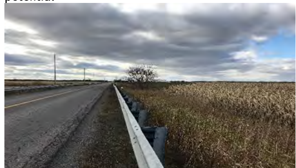
Plate 36: [SW] Burton Road; Area beyond disturbed ROW requires Stage 2
