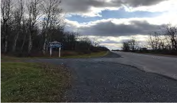
Plate 15: [SE] Boundary Road at Burton Road allowance; Area beyond disturbed ROW and ditch requires Stage 2
