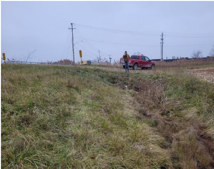
Photo 29: Disturbed ROW, built up and culverted, facing west
