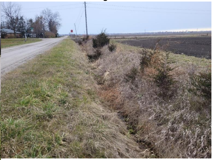
Photo 26: Ditched ROW, facing north
