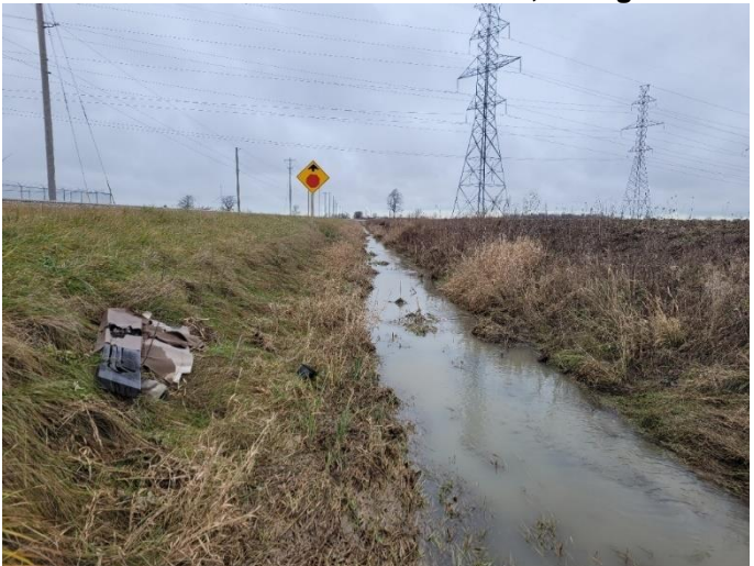
Photo 56: Deeply ditched ROW, facing north
