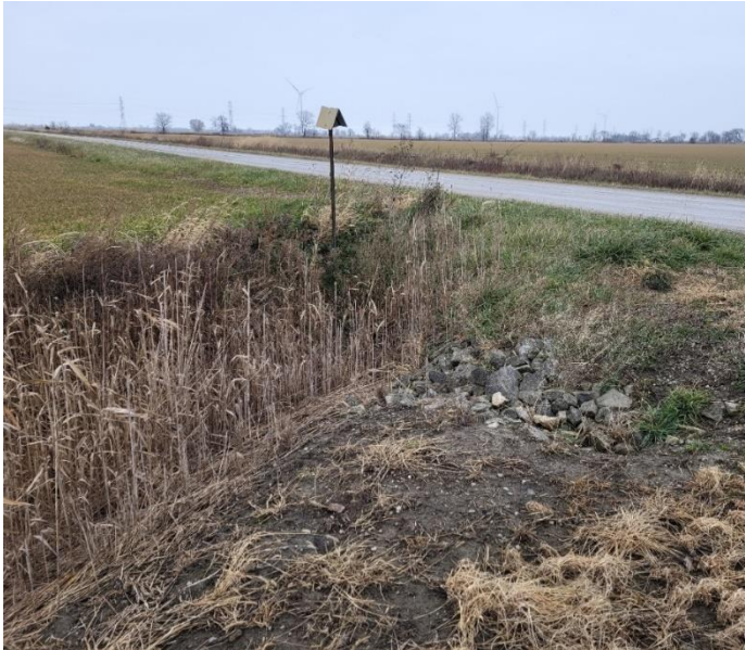
Photo 39: Ditched and culverted ROW, facing northeast
