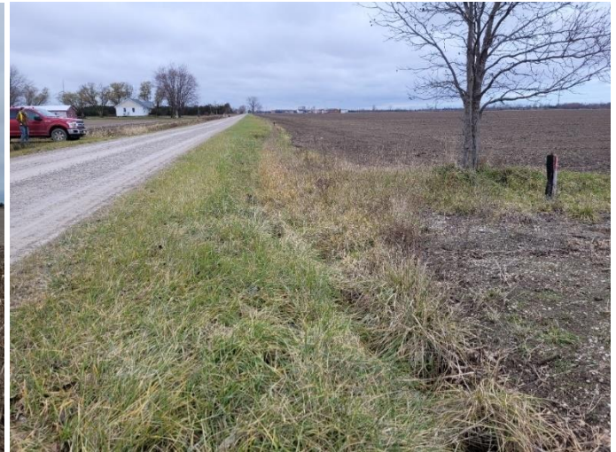
Photo 92: ROW disturbed and ditched, facing west
