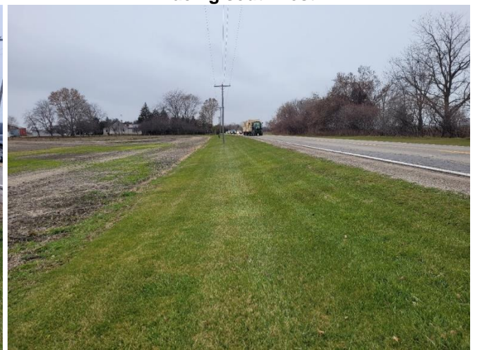
Photo 16: ROW graded to slope, facing west
