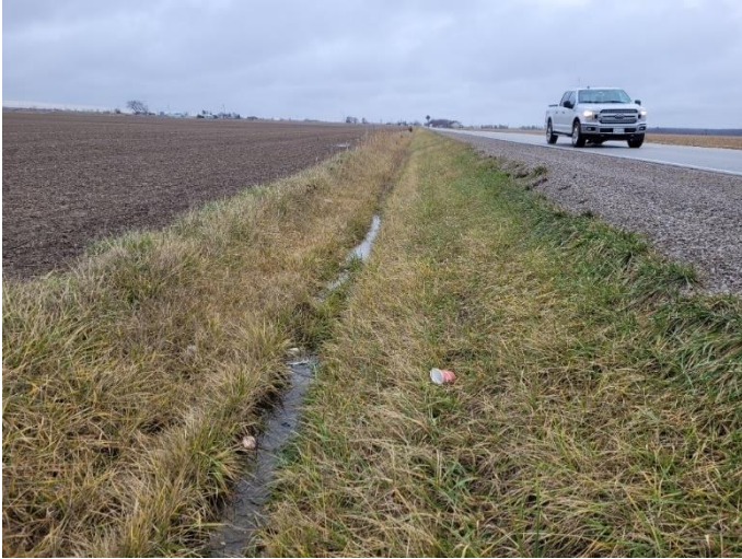
Photo 65: Ditched ROW, facing east
