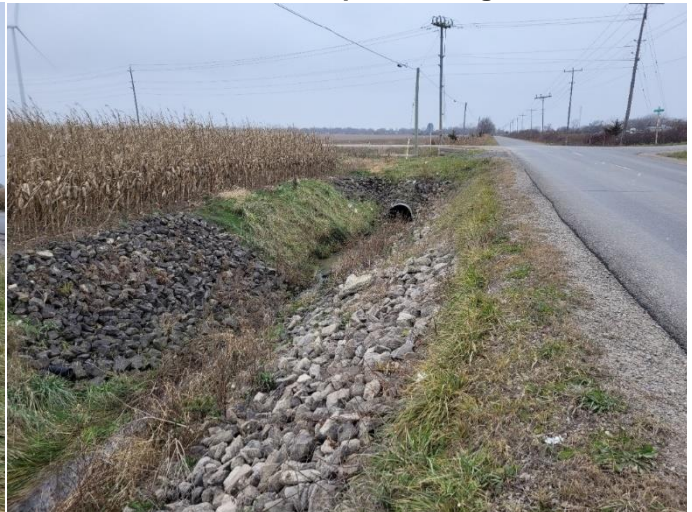
Photo 34: Deeply ditched/reinforced ROW, facing west
