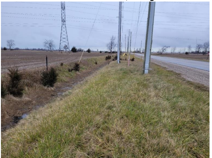
Photo 52: Deeply ditched ROW and utilities, facing north
