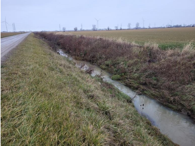
Photo 41: Deeply ditched ROW, facing northeast
