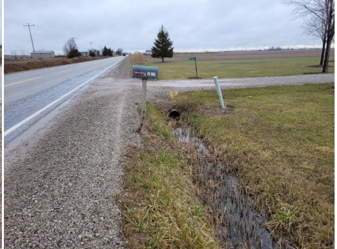
Photo 72: Ditched ROW with utilities visible, facing north
