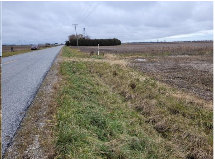
Photo 88: ROW, disturbed, ditched and culverted with utilities, facing west
