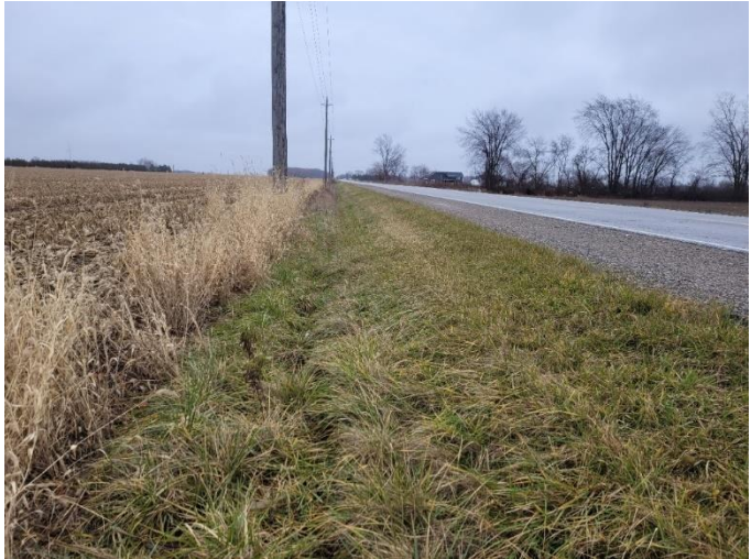
Photo 62: Ditched ROW, facing east
