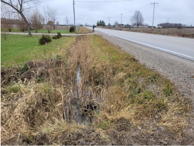
Photo 71: Deeply ditched ROW, facing south
