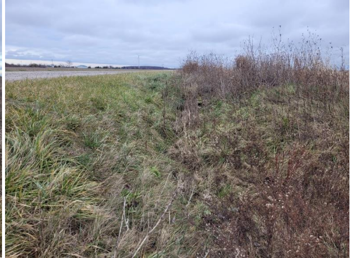
Photo 90: ROW, ditched and culverted, facing east
