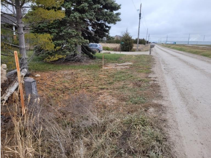
Photo 77: Disturbed ROW with utilities, facing east
