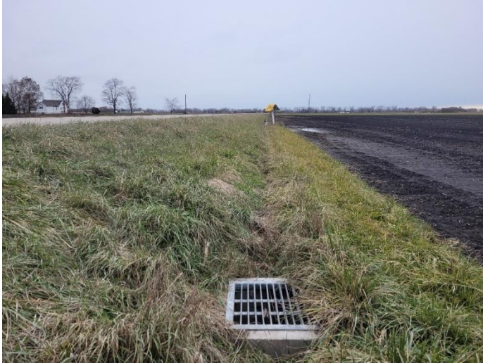
Photo 21: Ditched and disturbed ROW, facing north
