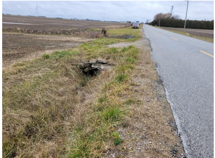
Photo 86: ROW, ditched and culverted, facing west
