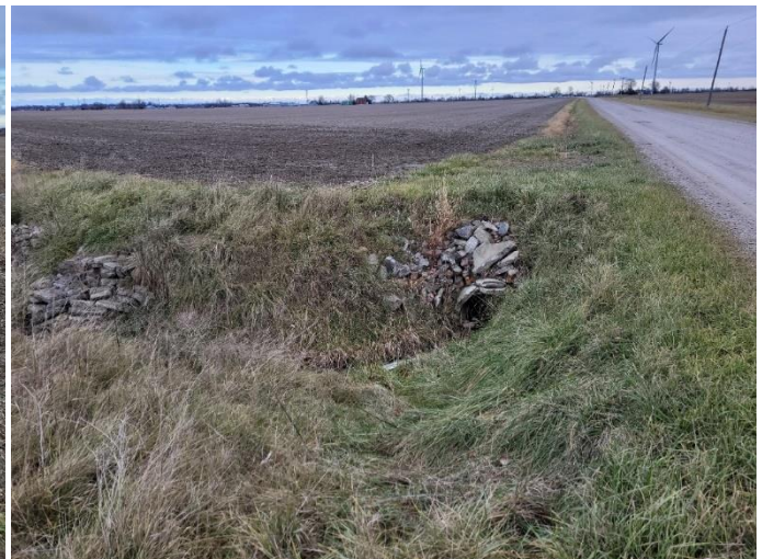
Photo 94: ROW, ditched and culverted, facing northeast
