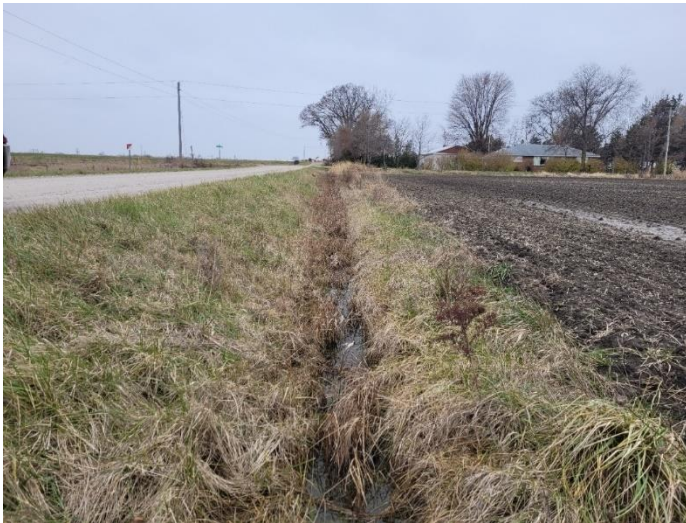
Photo 23: Ditched ROW, facing west
