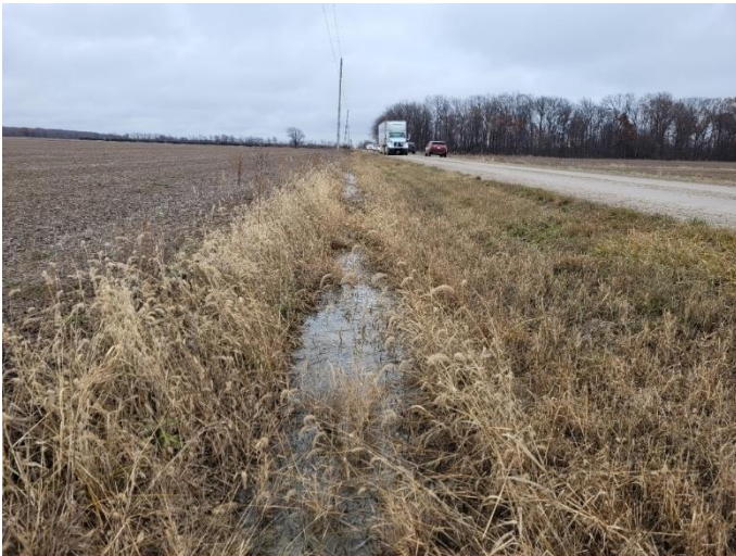
Photo 73: Ditched ROW, facing east
