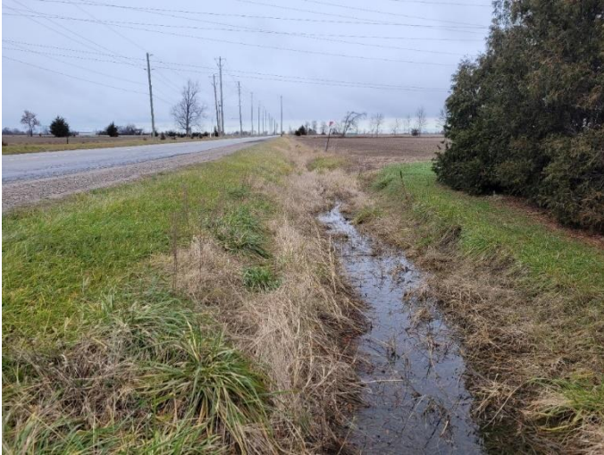
Photo 53: Ditched ROW, facing north
