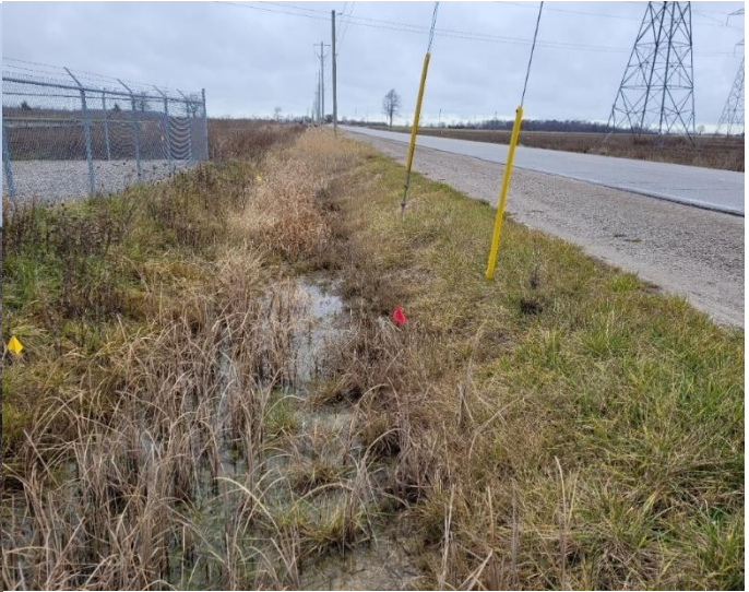
Photo 58: Disturbed ROW, ditched, utilities visible, facing north
