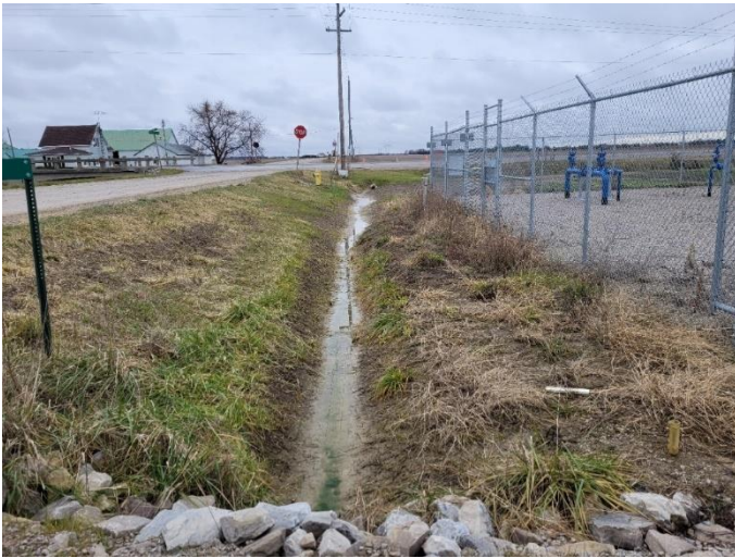
Photo 79: Disturbed ROW, ditched, utilities visible, facing west
