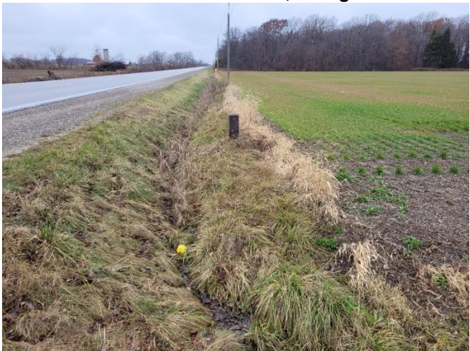
Photo 64: Ditched ROW with utilities visible, facing west
