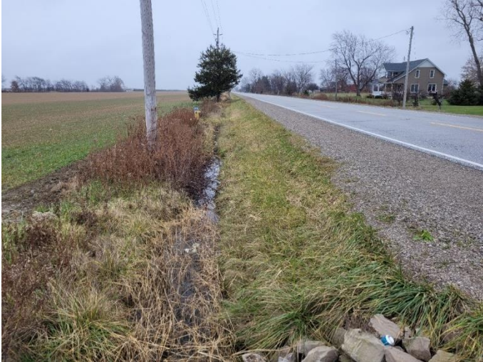
Photo 59: Ditched ROW, utilities visible, facing east
