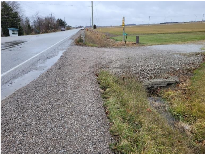
Photo 67: Ditched ROW, facing west
