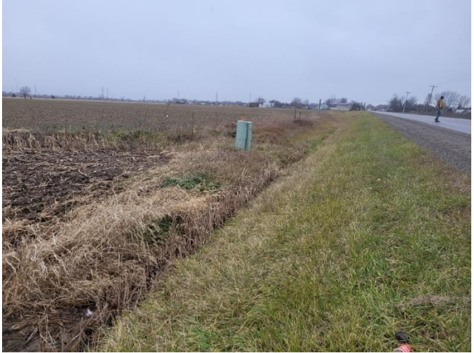
Photo 48: Ditched ROW, facing north
