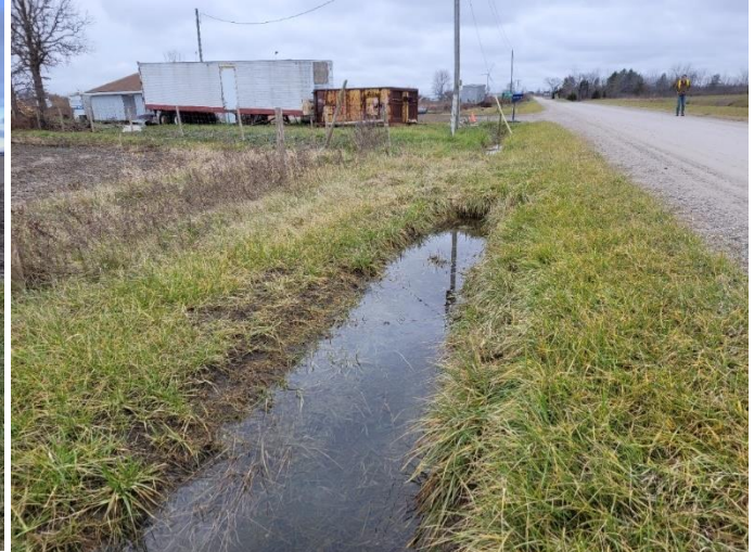
Photo 96: ROW, disturbed and ditched, facing west
