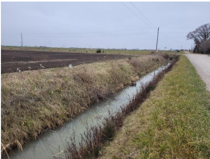
Photo 25: Deeply ditched ROW, and existing conditions in agricultural field, facing west
