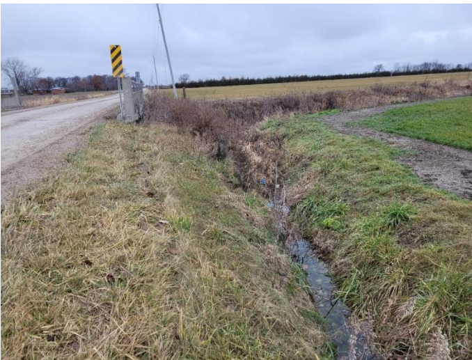
Photo 75: Ditched ROW, facing west
