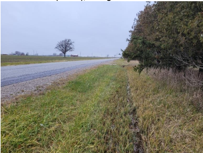
Photo 49: Ditched ROW, facing north
