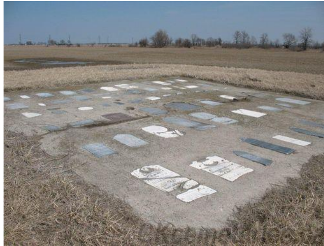
Plate 1: Malott cemetery concrete pad, demonstrating upright monuments encased in concrete for preservation (courtesy of John Skakel)
