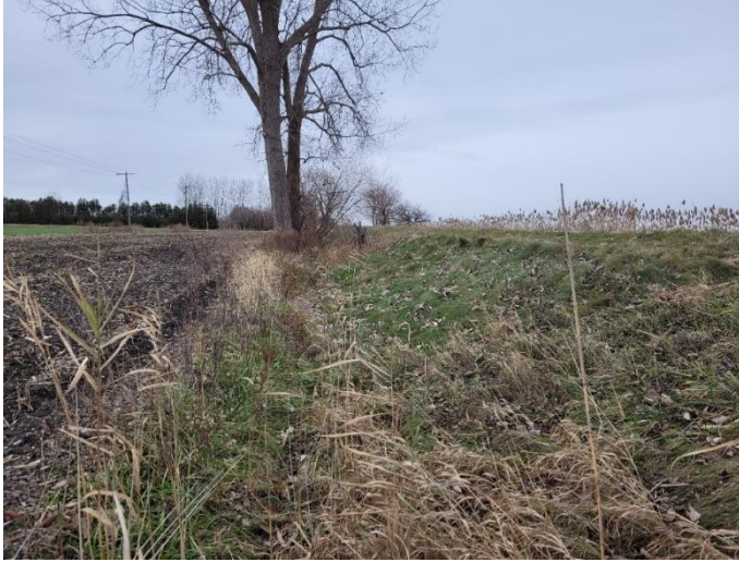
Photo 1: ROW disturbed, ditched and built up; facing southwest
