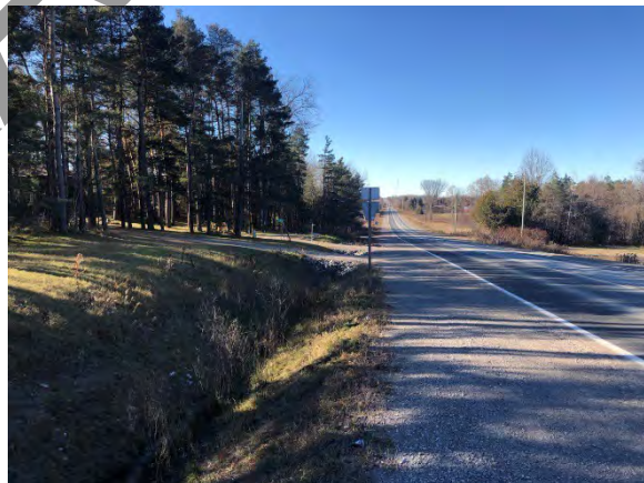
Photo 12: View of disturbed municipal road ROW, facing southwest
