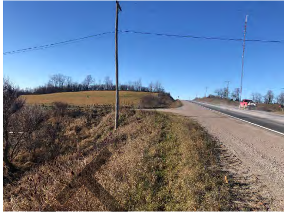
Photo 6: View of disturbed municipal road ROW, facing southwest
