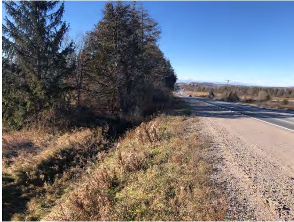
Photo 5: View of disturbed municipal road ROW, facing southwest
