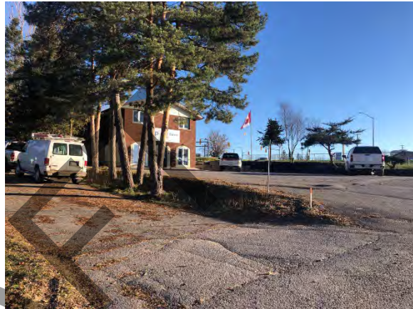
Photo 2: View of disturbed asphalt parking lot and building, facing southeast
