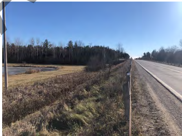
Photo 24: View of disturbed municipal road ROW, facing southeast
