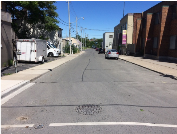
Photo 27: View of Labatt Avenue at River Street – disturbed, facing northeast
