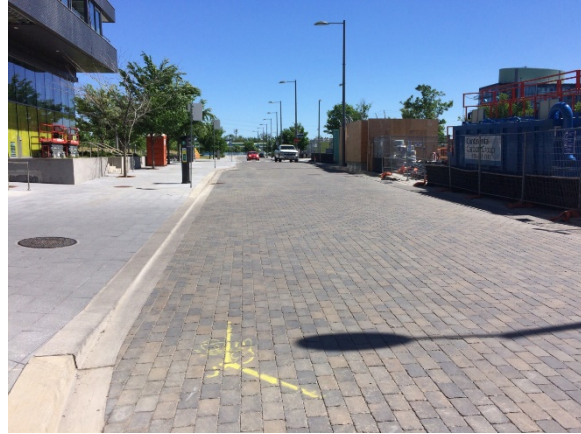
Photo 30: View of Tannery Road at Palace Street – disturbed, facing south
