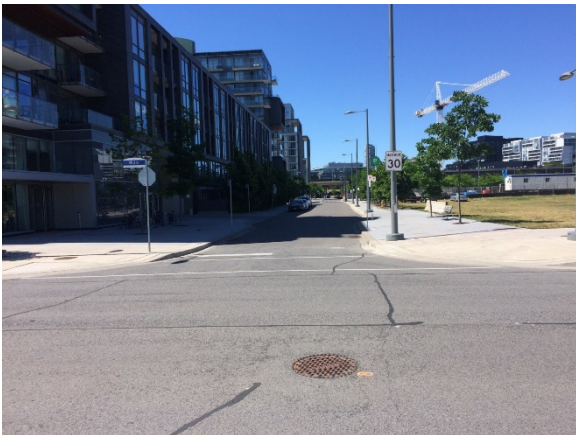
Photo 35: View of Rolling Mills Road at Mill Street – disturbed, facing north
