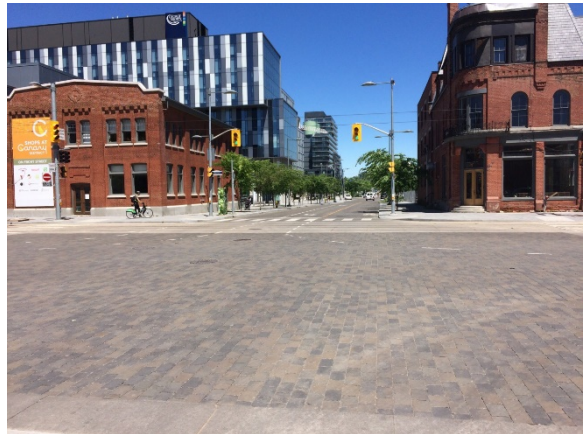
Photo 8: View of Front Street East at Cherry Street – disturbed, facing northeast
