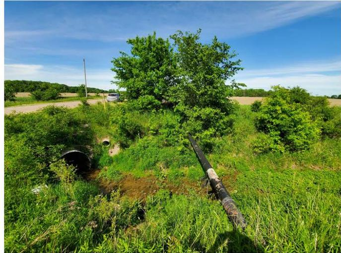
*Figure 8: Aerial Crossing with pipe coating peeling off (Falconbridge, between Tait's Rd and McArthur Rd). Left is a close-up, right show the crossing in context.*
