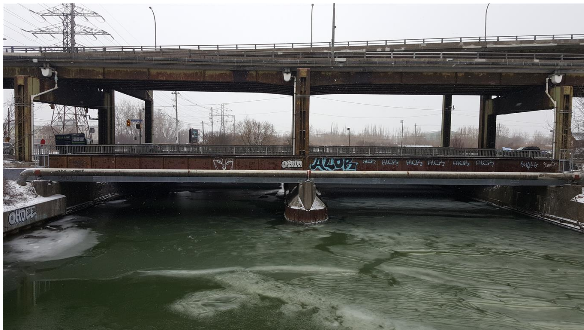
Figure 2. Keating Railway Bridge (from pedestrian bridge looking downstream)
