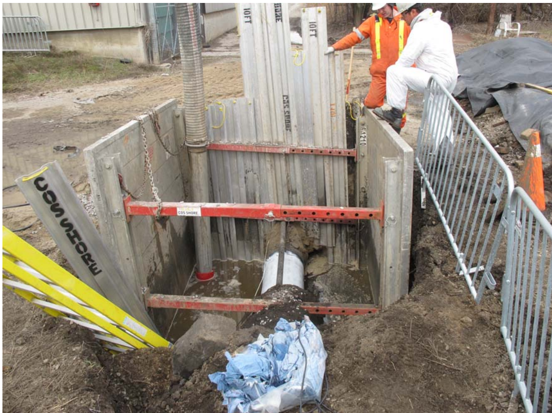
02 - Exposed areas NPS 20 in KOL LINE
