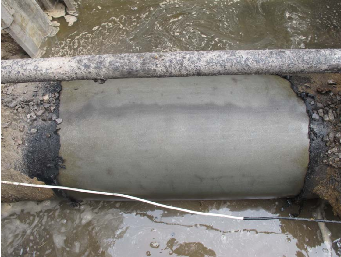
03 - Pipe found in good condition
