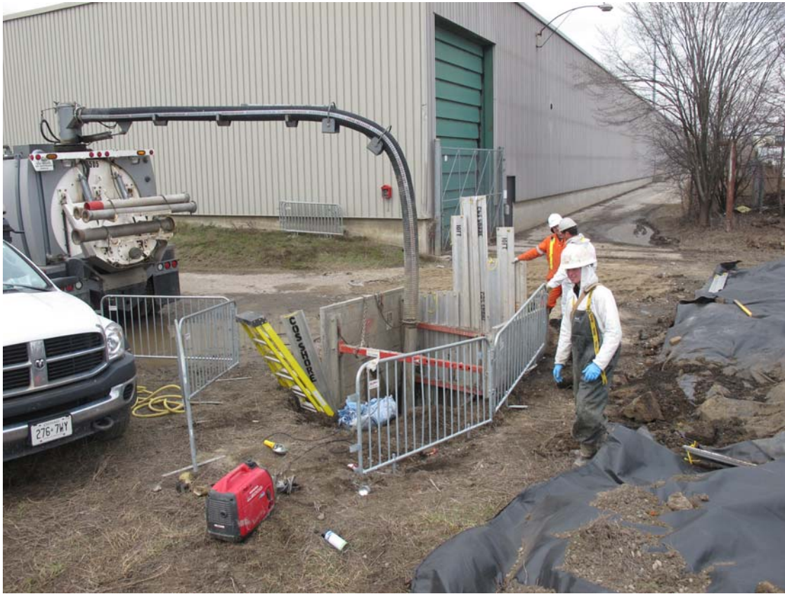
01 - Site location facing downstream
