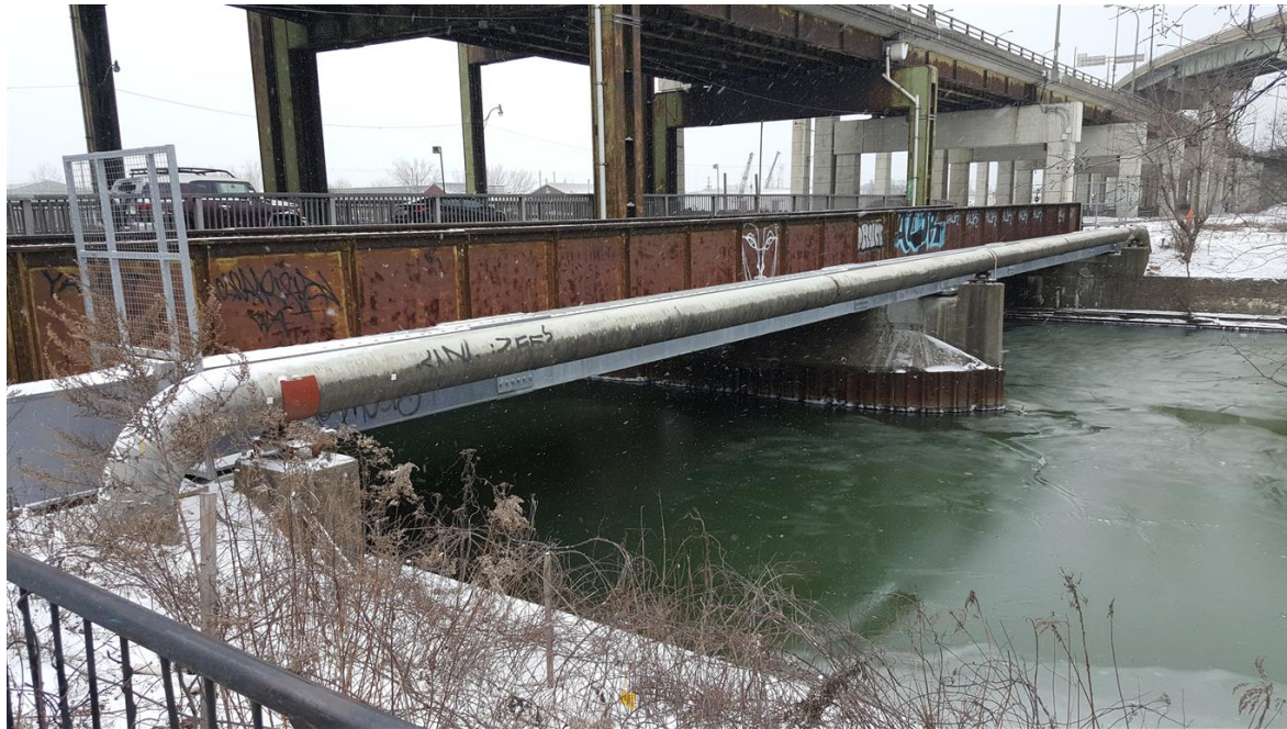
Figure 1. Keating Railway Bridge (from left bank)
