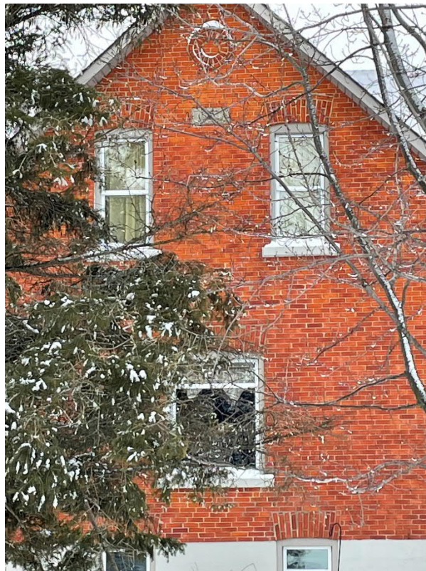
Photograph 4: Close-up of 23696 Dashwheel Road showing brick voussoirs and circle details (AECOM 2022)
