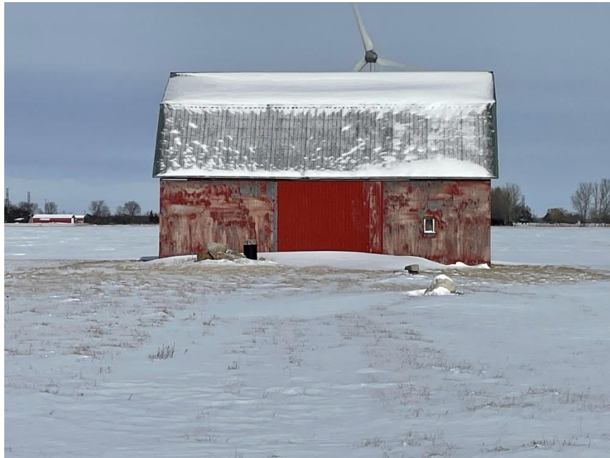
Photograph 12: Close-up of remaining barn at 19800 Desimpel Road (AECOM 2022)
