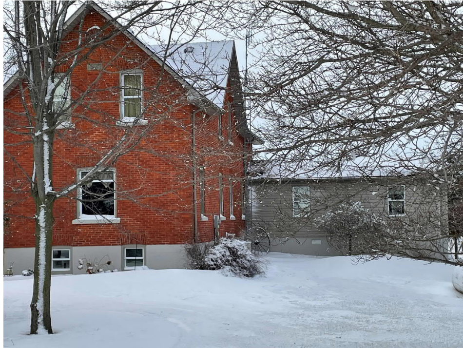
Photograph 3: 23696 Dashwheel Road showing brick structure and one-storey addition (AECOM 2022)
