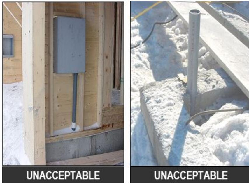
**Left:** The PVC conduit extends more than 300 mm (12 in.) above the base of the foundation. This type of installation requires additional consideration and approval by the Enbridge Gas Engineering department before construction starts (i.e., when submitting a preliminary request for site servicing).
