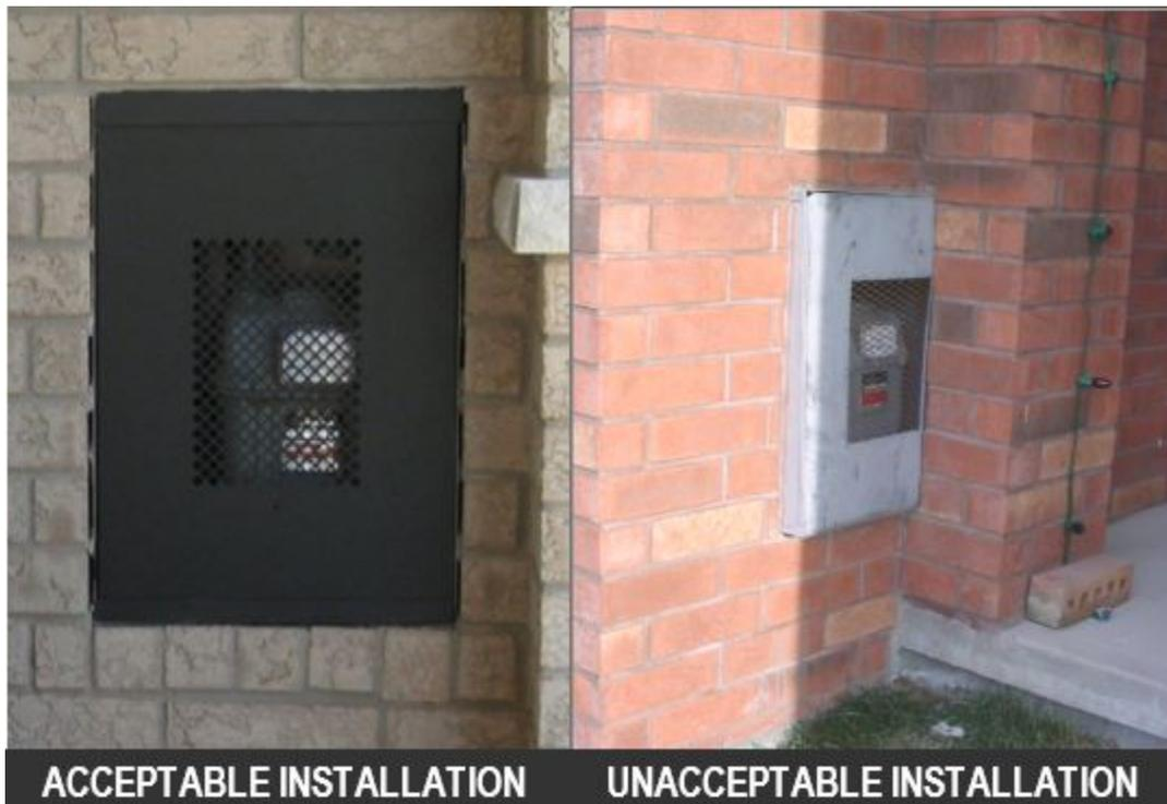
**Left:** An acceptable installation incorporates the following: a secured box (sitting on foundation or otherwise secured), use of lintel angles, sufficient clearance from openings, and a door which opens freely (not fixed or nor tampered).
