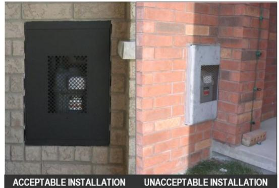
Figure 5-2: Examples of acceptable and unacceptable meter box installations
