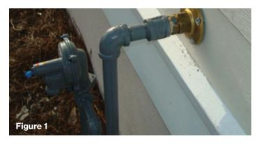
These techniques will provide adequate support for the meter without the requirement of piping supports.
