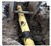
Figure 5.2-25: Gouges and dents due to latent damages
