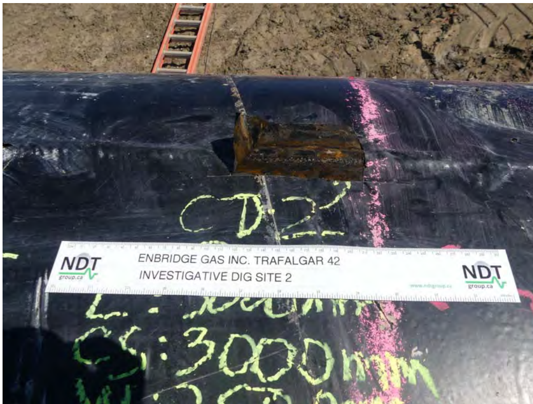
021 - CD-02 COATING REMOVED BLACK, ORANGE CORROSION DEPOSIT
