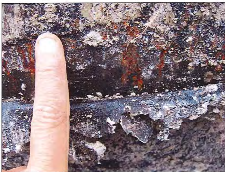
Photograph 5-3 • Site #1. Sample of Coating Damage. Ch. 68.45m (540cm)
