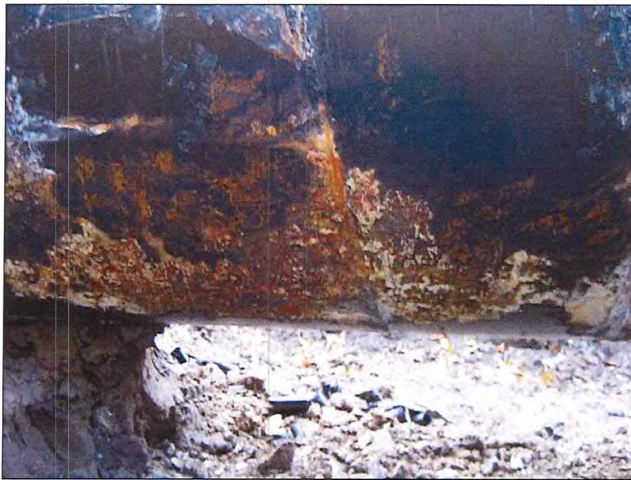
Photograph 7 • Site 1. General Corrosion and Calcareous Deposits.
