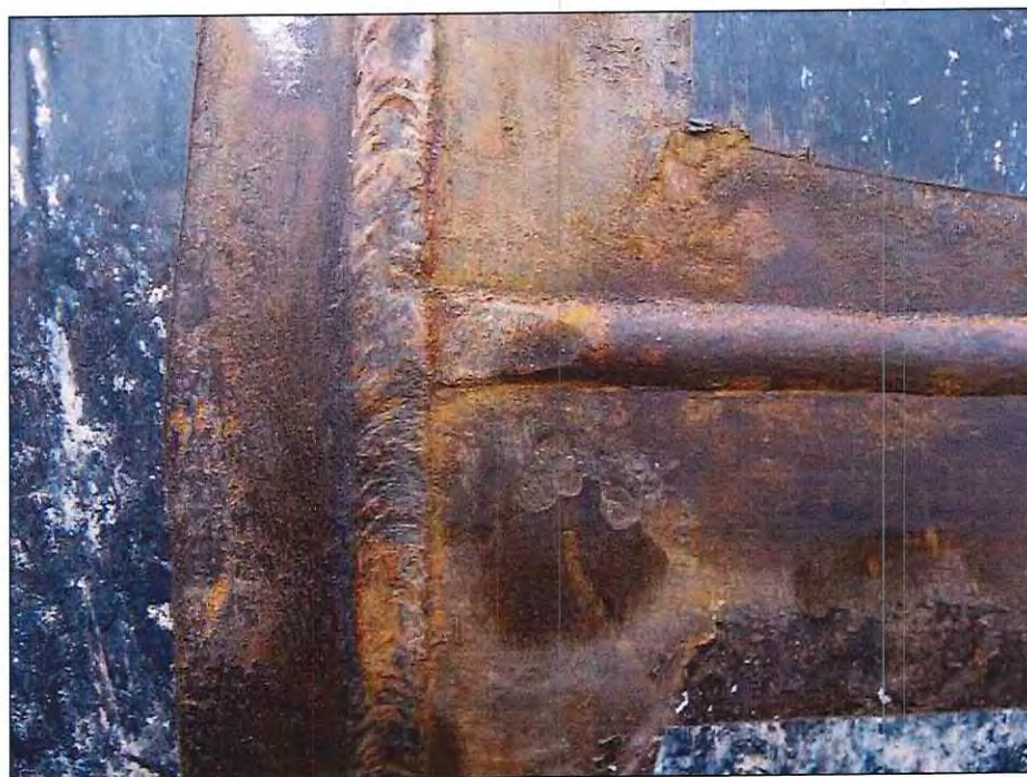
Photograph 22 • Site 2. Pipe Exposed at Girth Weld.
