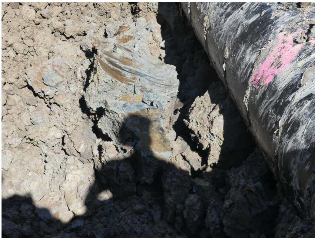
007 - STRONG GLEYING WAS FOUND AT BOTTOM OF PIPE
