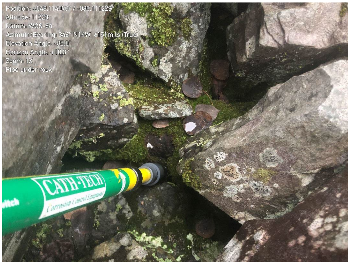
Figure 5: Exposed Pipeline Under Rock Boulders
