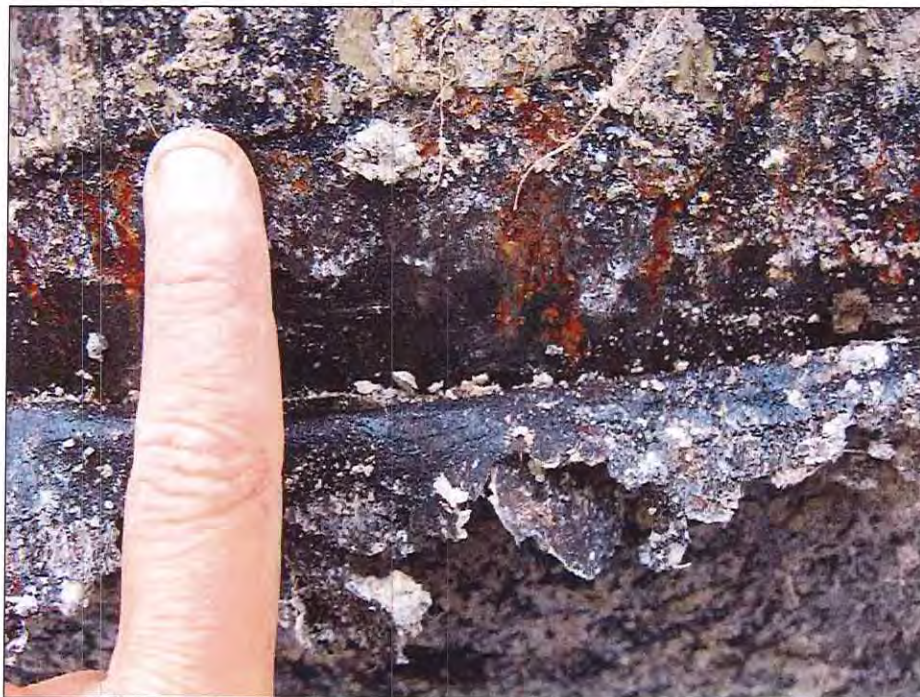
Photograph 3 • Site 1. Sample of Coating Damage. Ch. 68.45m (5.40m).
