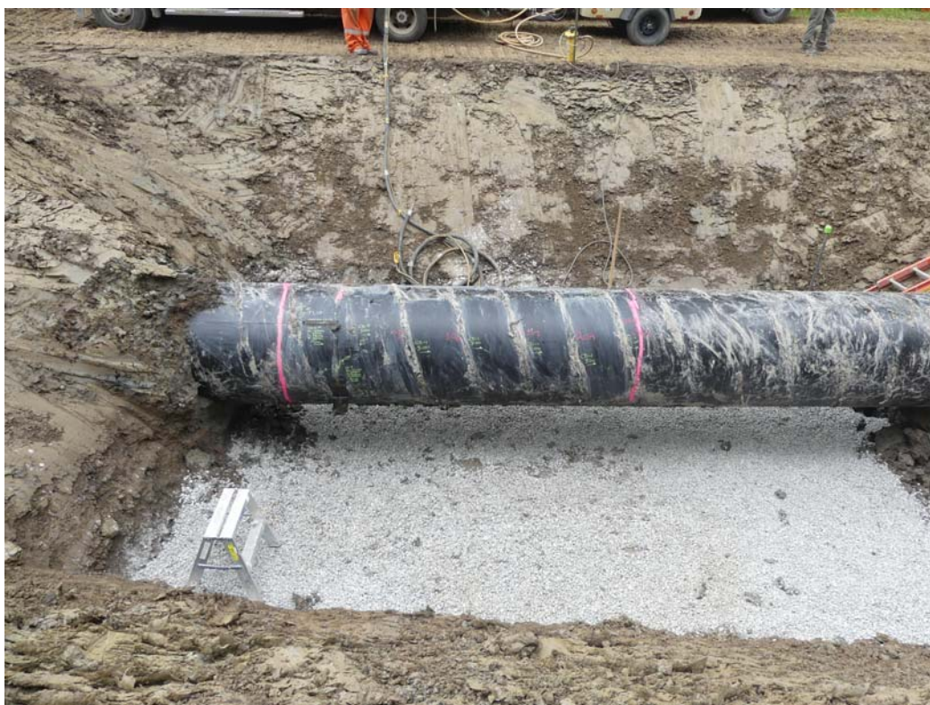
008 - COATING ASSESSMENT AREA 3 O'CLOCK SIDE
