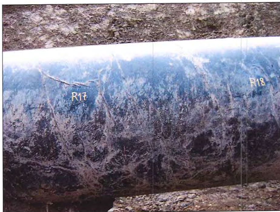
Photograph 13 • Site 2. Disbonded Coating at Longitudinal Weld. Looking South – 03.
