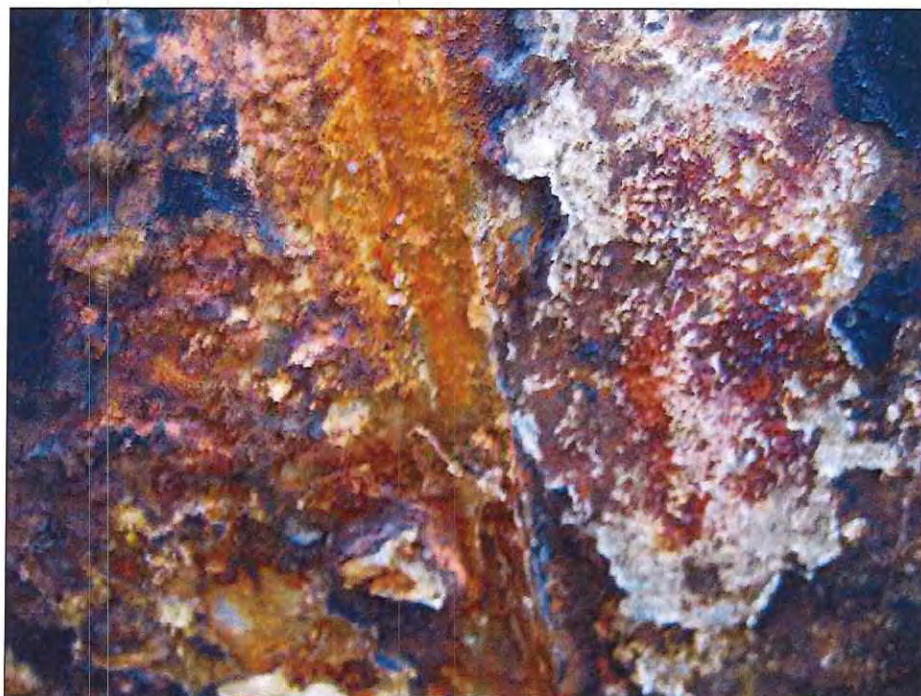
Photograph 8 • Site 1. General Corrosion and Calcareous Deposits. Close View.
