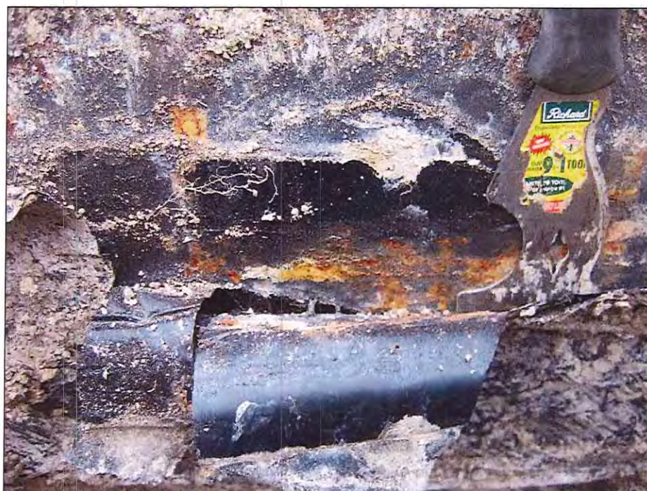
Photograph 4 • Site 1. Sample of Coating Damage. Ch. 69.45 (6.40m).
