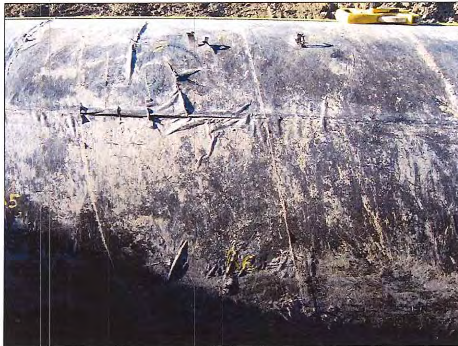
Photograph 7 • Site 2. Disbonded Coating at Longitudinal Weld. Looking North – 05.
