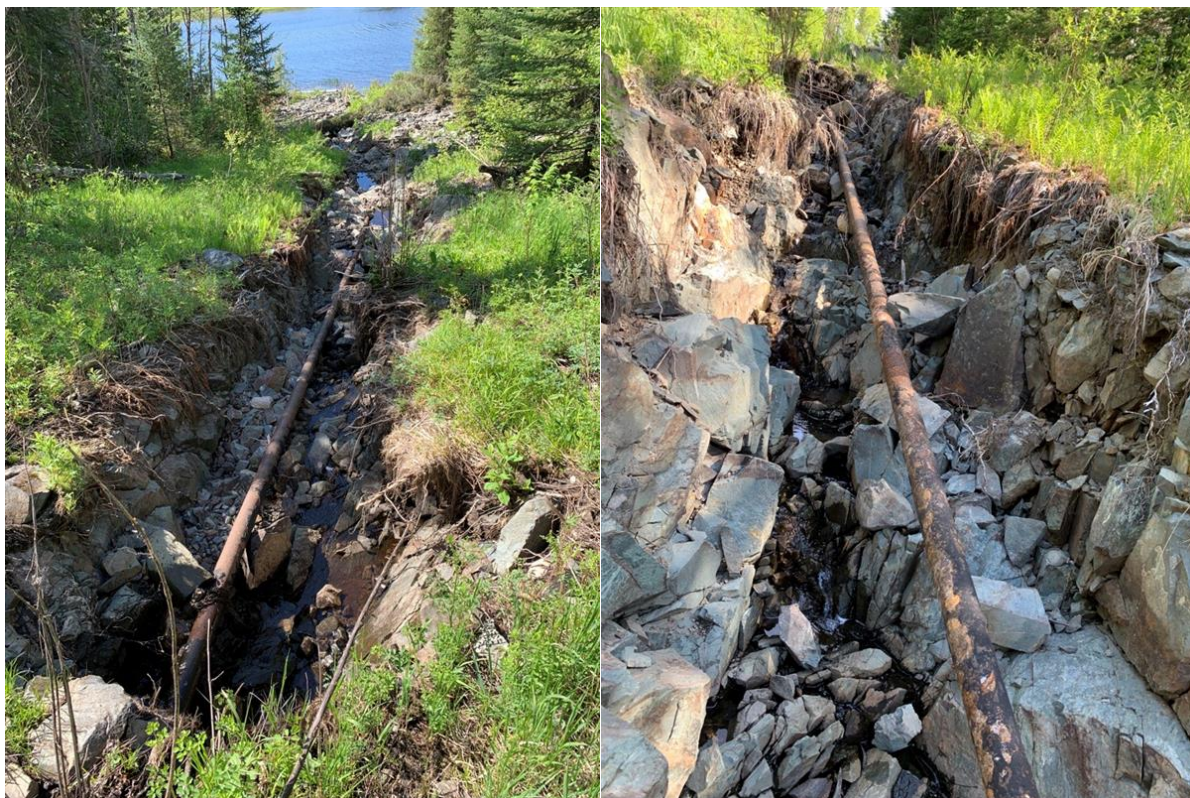
Figure 4: Washout of the Existing Line
