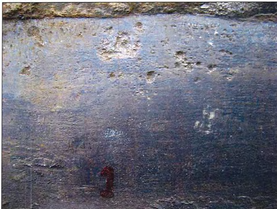
Photograph 24 • Site 2. Sample of Shallow Pit (R12 – Pit #1).
