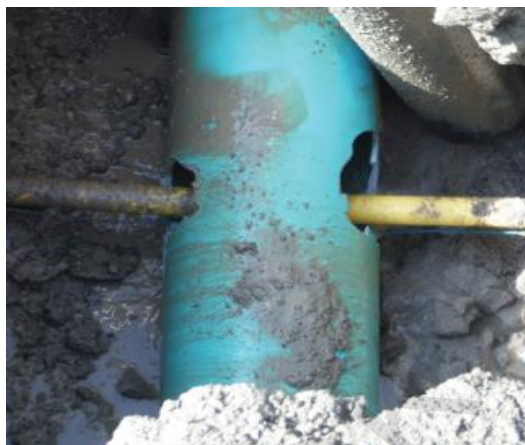
Image: Example of a cross bore
