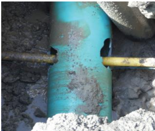
Image: Example of a cross bore
