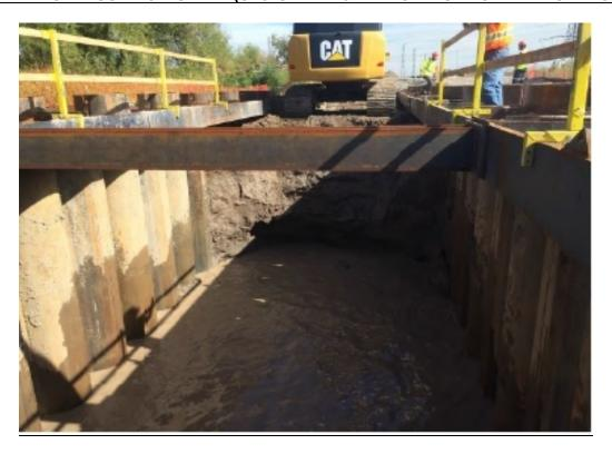
REDACTED Filed: 2002/3-063308/GEB-12/06/32:0-21906;t Extristitulation 12F-56/Encial 2R-4/tarch/Appendix B-algerge-32-6 for 50 LISGAR MEADOWBROOK (BOILING SAND FLOWING THROUGH SHEET PILING)
