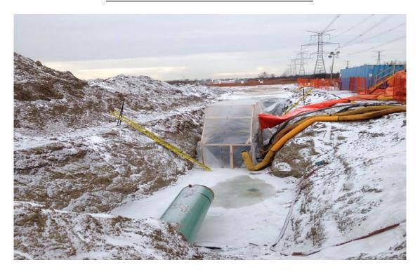
SEDIMENT FILTRATION FOR DISCHARGE WATER AT KENNEDY ROAD TEST SITE
