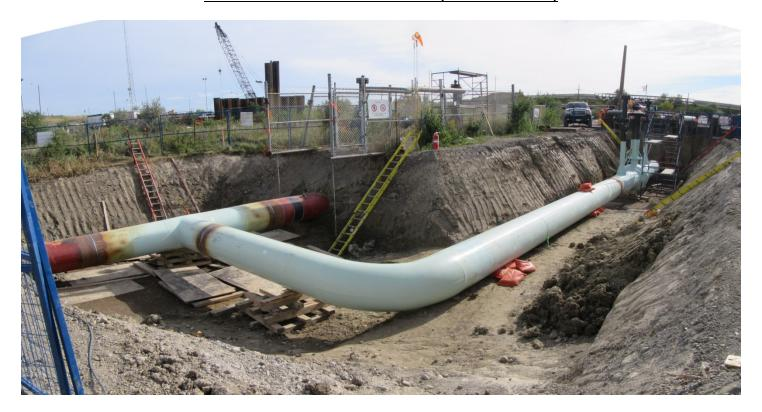
NPS 36 CN TRACK BORE TO ALBION STATION (NORTH SIDE PIT WITH PIPE INSTALLED & SOUND CURTAIN)
