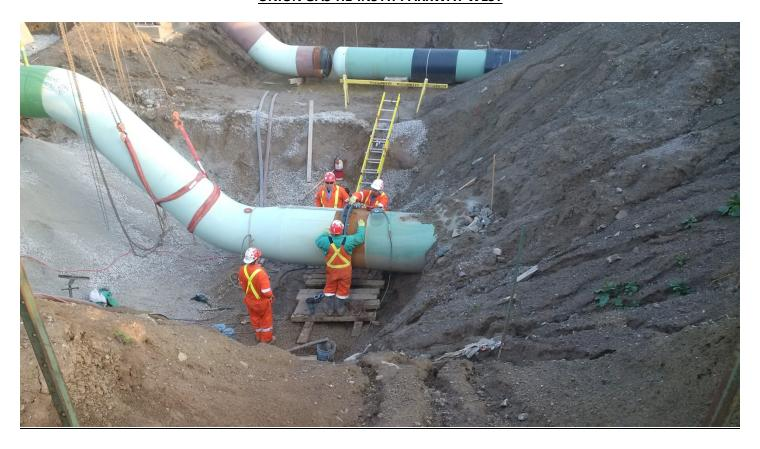
NPS 42 PIG LAUNCHER BEING LOWERED INTO PLACE AT PARKWAY WEST
