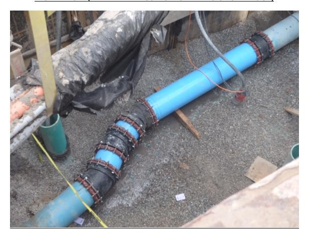
LISGAR MEADOWBROOK EAST BORE PIT (UNSTOPPABLE SAND FLOWING INTO PIT LED TO DIRECT PIPE)
