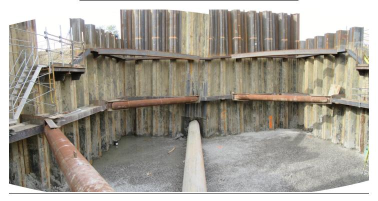
CONSTRUCTION OF L-SHAPED NPS 42 CN TRACK BORE PIT (NORTH SIDE TO TIE IN OF FINCH-CLAIREVILLE HDD)
