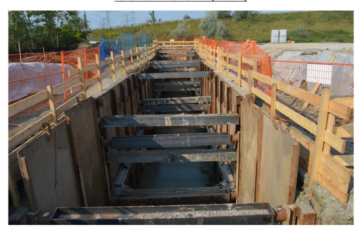
**BEAVER CREEK TRIB 2 (INSTALLING CONCRETE COATED PIPE)**
