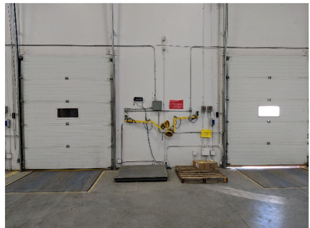
Loading Dock (top): A typical loading dock with bumpers, dock levelers, shroud, and red/green traffic light. (bottom) Two drive-on loading docks, with insulated metal panels and a single vision panel.
