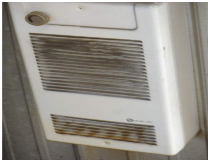
2. Electric Unit Heater
