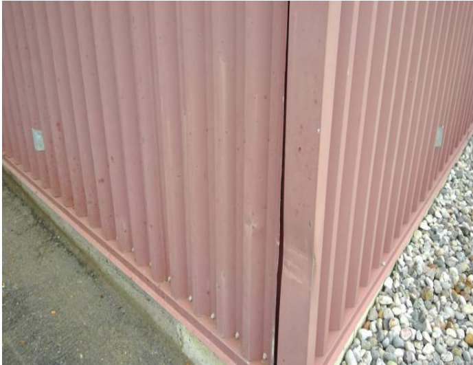
3. Deteriorated Metal Cladding
