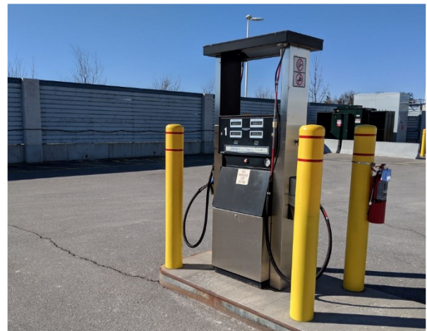
NGV Fill Stations: Operations Centres may be designated to have on-site natural gas fueling stations to support their fleet. The station consists of a compressor and a pump station with card access. Basic NGV layout principles are covered in 4.1.6 NGV Fill.
