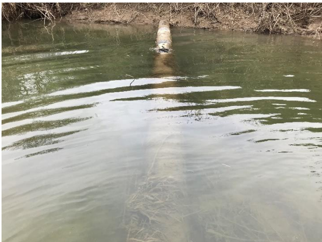
Photo 5: Exposed length of pipe
