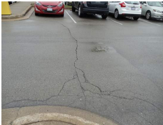
1. Cracked Asphalt
