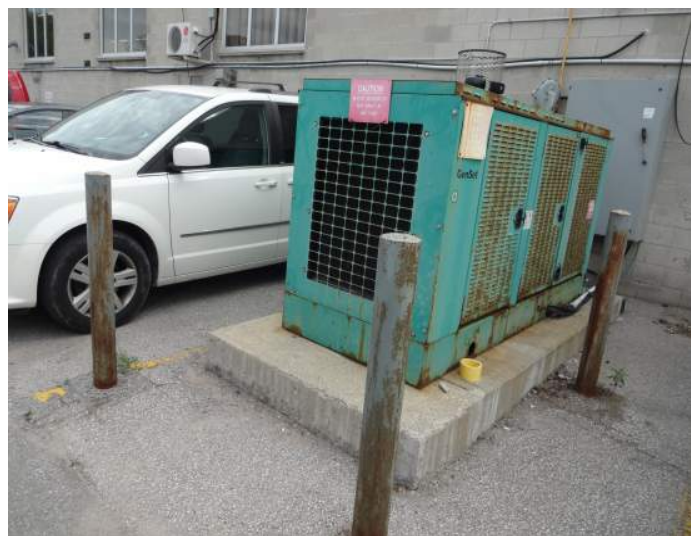
4. Generator Requiring Replacement
