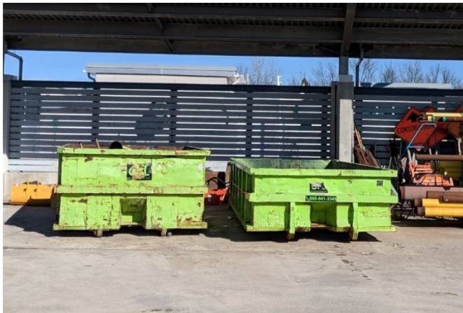
Waste Bins: Standard waste and miscellaneous waste bins should be in easily accessible areas. Ensure appropriate space is given for truck access.
