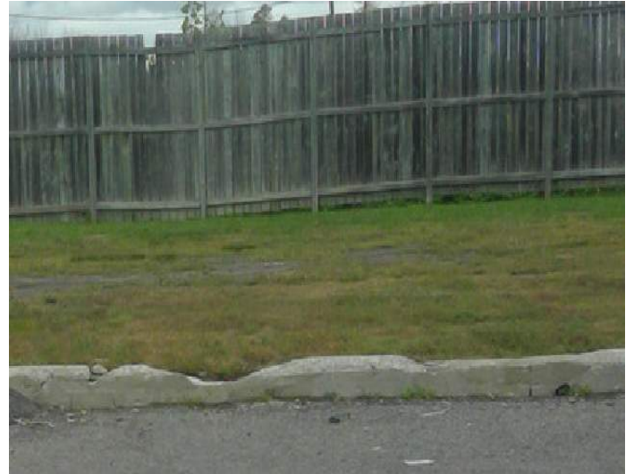
4. Wood Fence and Curb Deterioration
