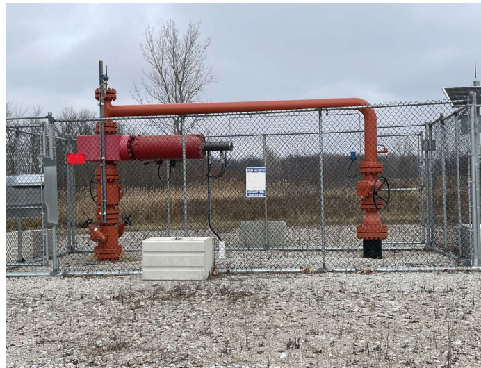
Image 1. Typical Injection – Withdrawal Well Wellhead
