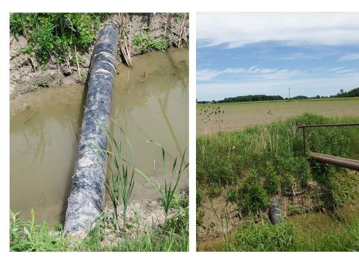
Figure 6: Aerial Crossing and bridge used for inspection, prone to partial submersion (Pratt Siding and Knapdale, through private easement). Left is a close-up, right show the crossing in context.
