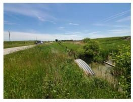
Figure 5: Aerial Crossing near municipal drain, potential for pipe to be partially submerged (Mosside Line, West of Burr Rd). Left is a close-up, right show the crossing in context.
