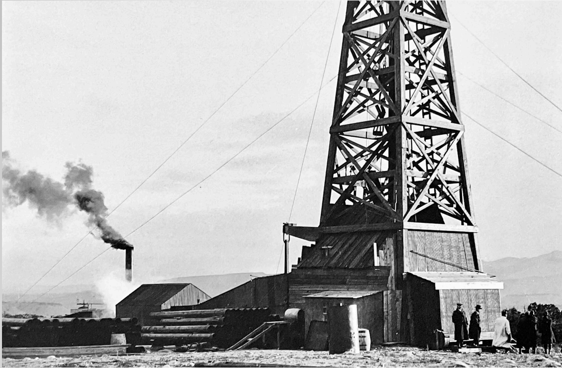
Steam-powered cable-tool drilling rig circa 1921.
