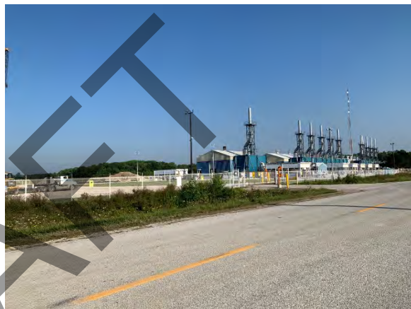
Photo 2: View of existing Enbridge infrastructure within the study area, facing northwest
