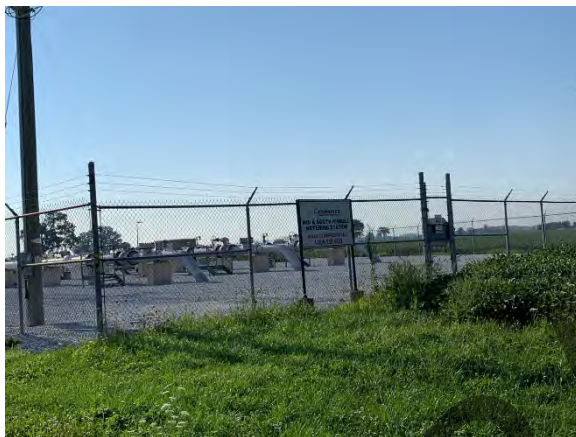
Photo 1: View of existing Enbridge infrastructure within the study area, facing southeast
