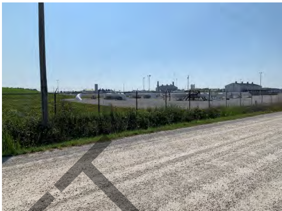
Photo 26: View of existing Enbridge infrastructure within the study area, facing southeast
