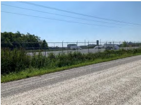
Photo 25: View of existing Enbridge infrastructure within the study area, facing southeast
