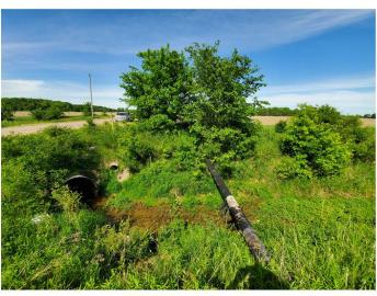
Figure 8: Aerial Crossing with pipe coating peeling off (Falconbridge, between Taits Rd and McArthur Rd). Left is a close-up, right show the crossing in context.
