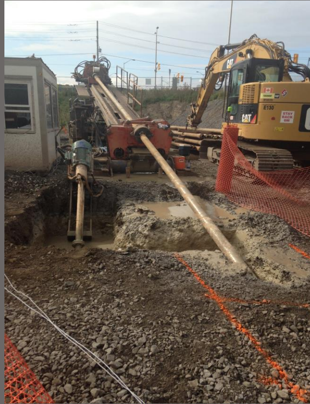
Example of Horizontal Directional Drilling work on a similar project.
