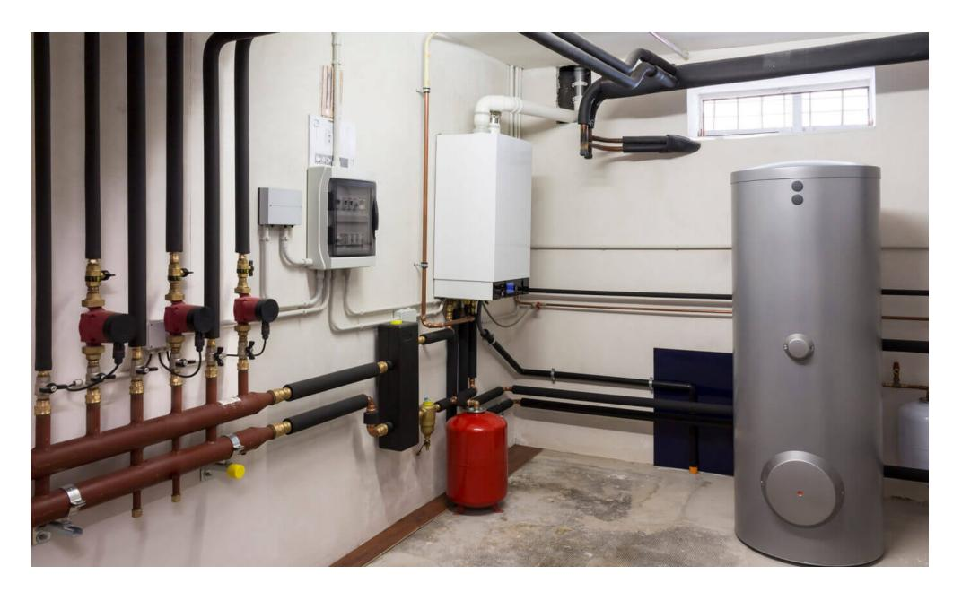
First, let's review Boiler 101: A boiler works by extracting heat from the fuel it burns. In both high-efficiency and condensing boilers, that heat is first pushed through a heat exchanger, which transfers energy to the water that runs through radiators and baseboards.
