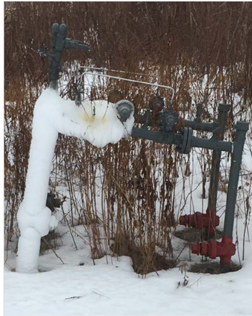
Figure 5.3-10: The Joule-Thomson Effect on a District Station
