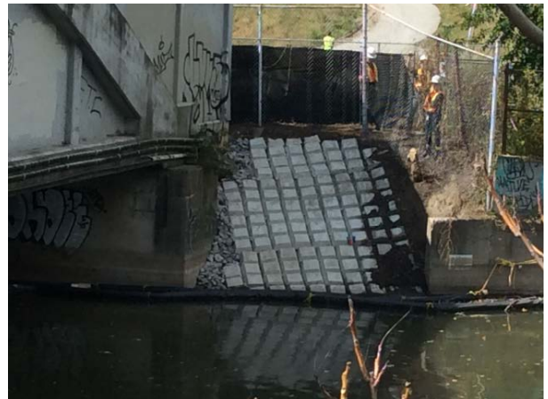
Figure 5.2-20: Temporary Remediation to the Undermined Abutment
