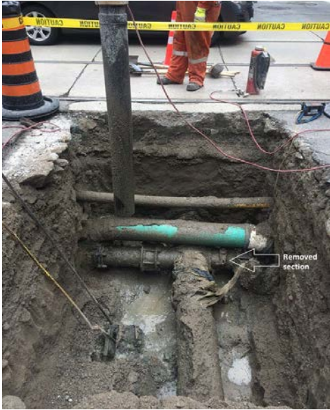
Figure 5.2-14: Leak Investigation on Vintage NPS 12 Gas Main
